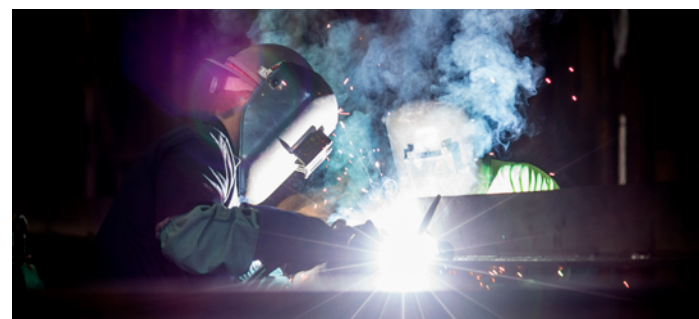
Welding requires specialized equipment and skill set
