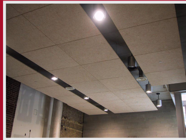
Panel and Ceiling Hanging
